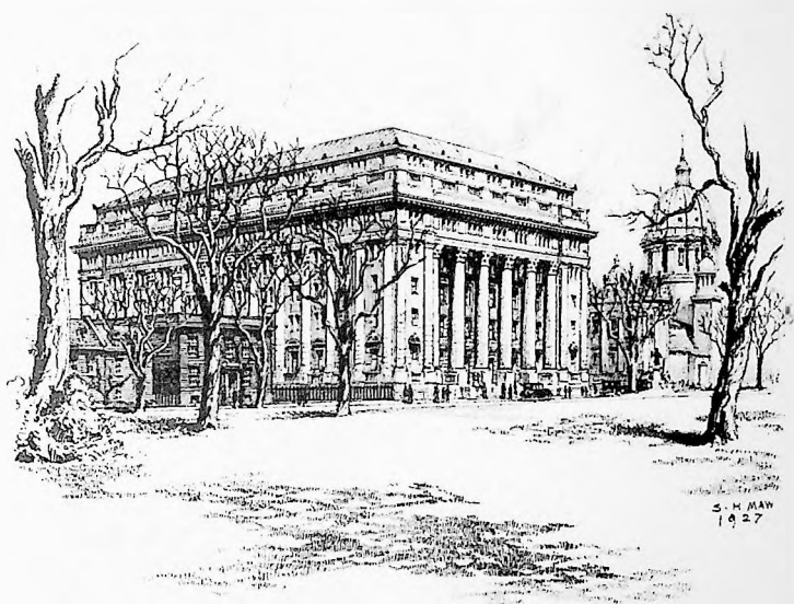
HEAD OFFICE BUILDING, MONTREAL
